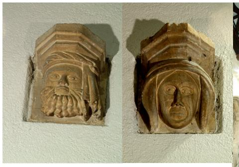
The carved head corbels would have originally supported the roof cross members which are the medieval originals. The roof tracery is, however, Victorian.
