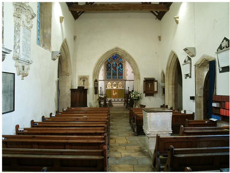
The nave shows the roof line has been raised as the corbels now sit isolated towards the top of the wall.
